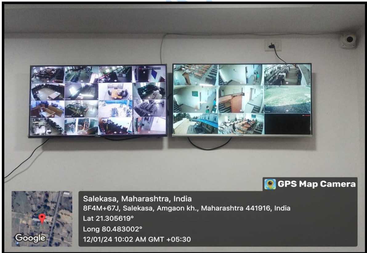
24 hr. CCTV Vigilance (total 24 camera)
