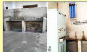
Ro Plant & Water Cooler
